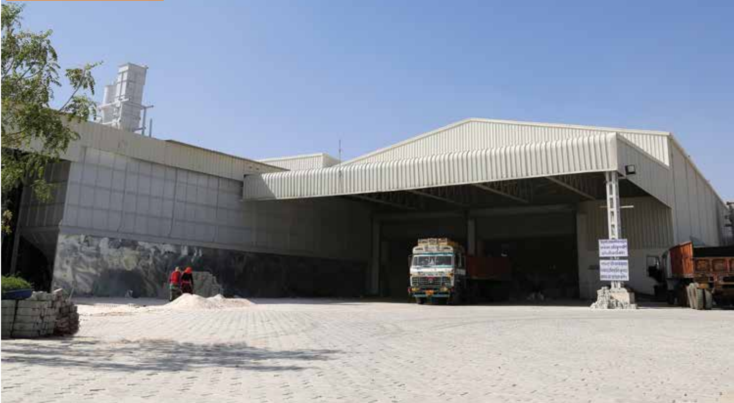
Ramming Mass Plant Loading Area
